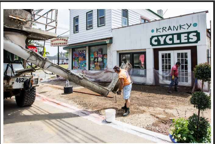
The Streetscape Phase I, continues on Waterwitch Ave.
