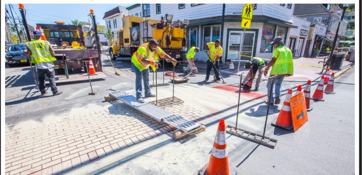
Streetscape cross walks installed in 2016
