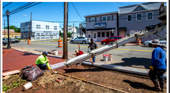
The Streetscape Phase II, began in 2016.
